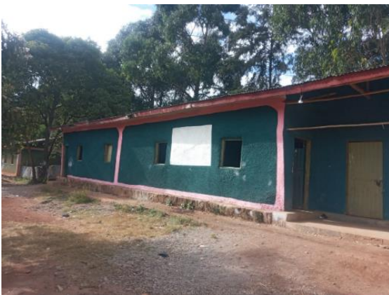
rooms and side view of the girls pit latrine
